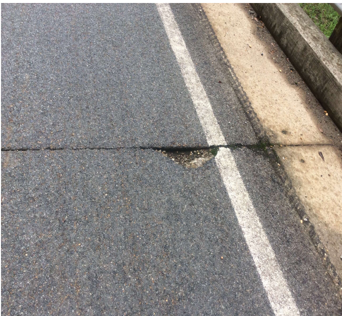
PHOTO 1 Description Deck - Bent 4 right. Pothole
